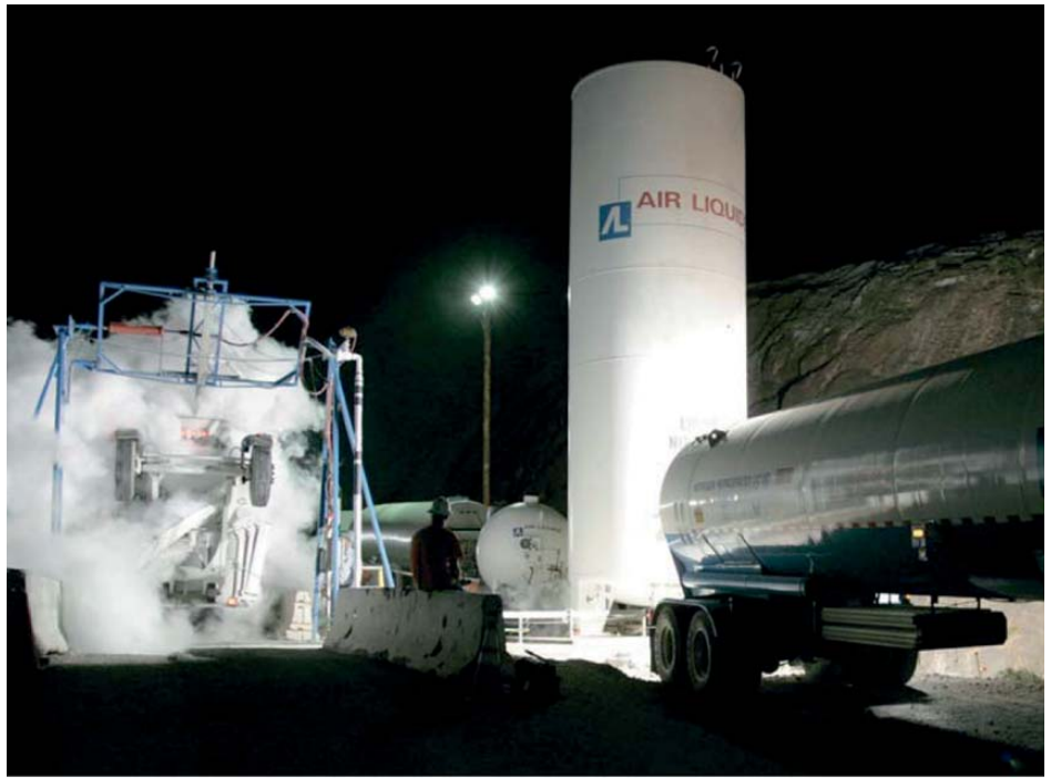
Airgas and Air Liquide use CryoCrete™ technology to inject liquid nitrogen into a redi mix truck to ensure optimal pour temperatures.
